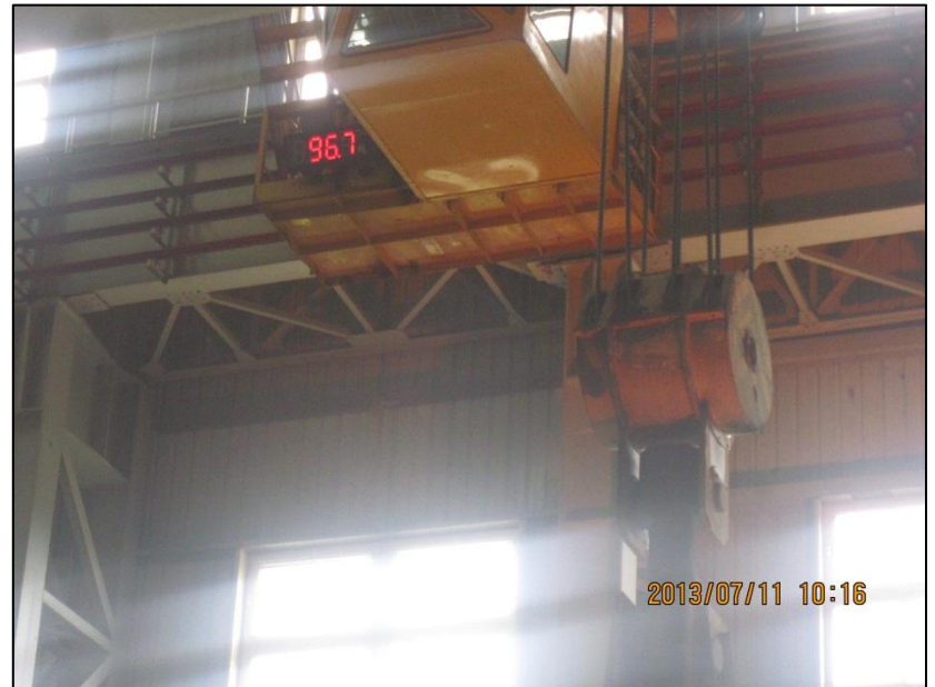
Crude Fe-Ni weighing
