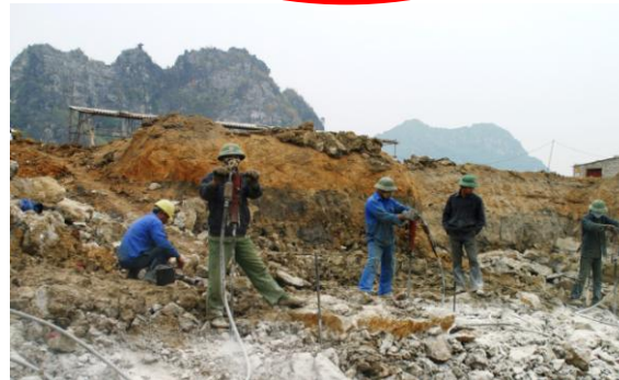
Blasting for digging foundations
