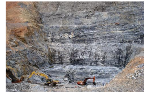
Blasting for digging foundations at new hydroelectric plants
