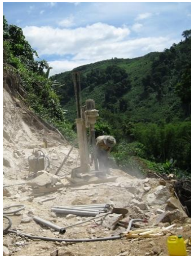
Blasting for road construction
