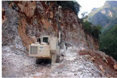
Blasting for road construction
