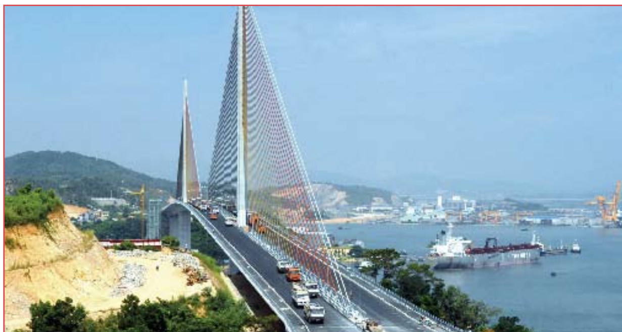
Bai Chay Bridge (supported by Japanese ODA)
