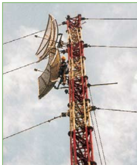
Checking a microwave station
