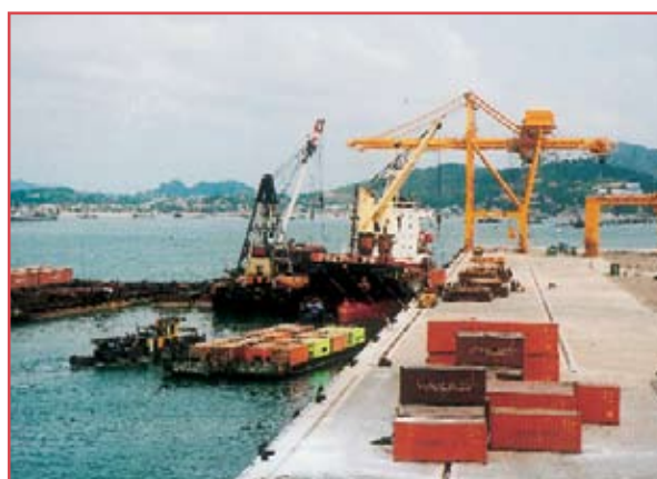
Cargo loading at sea port
