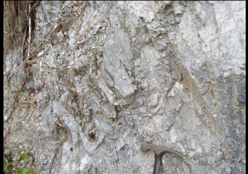
Crushed limestone within the Kisap thrust fault zone.
