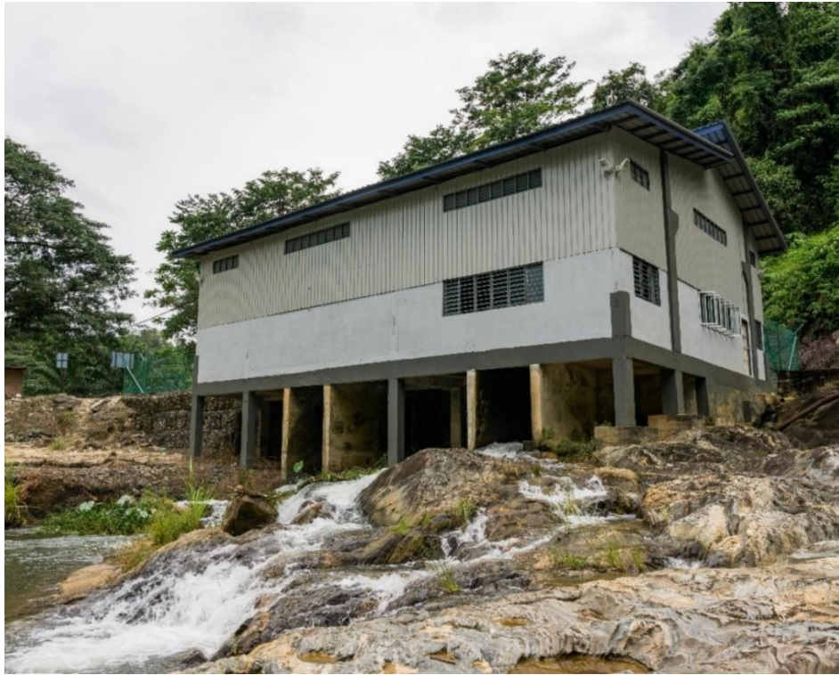
Figure 35: (Top) Cascading waterfall of Sungai Renyok. (Below) Hydroelectric station powered by Sungai Renyok.
