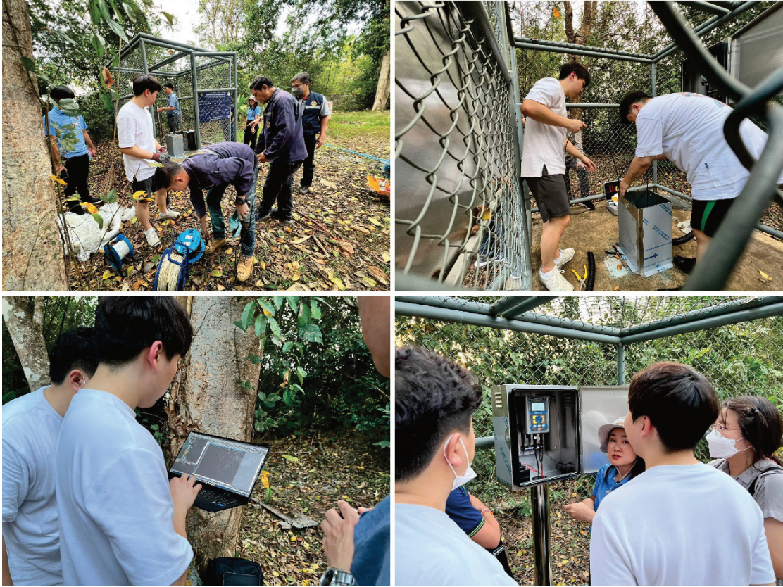
Groundwater monitoring system installation in Nakhon Phanom province, NW Thailand
