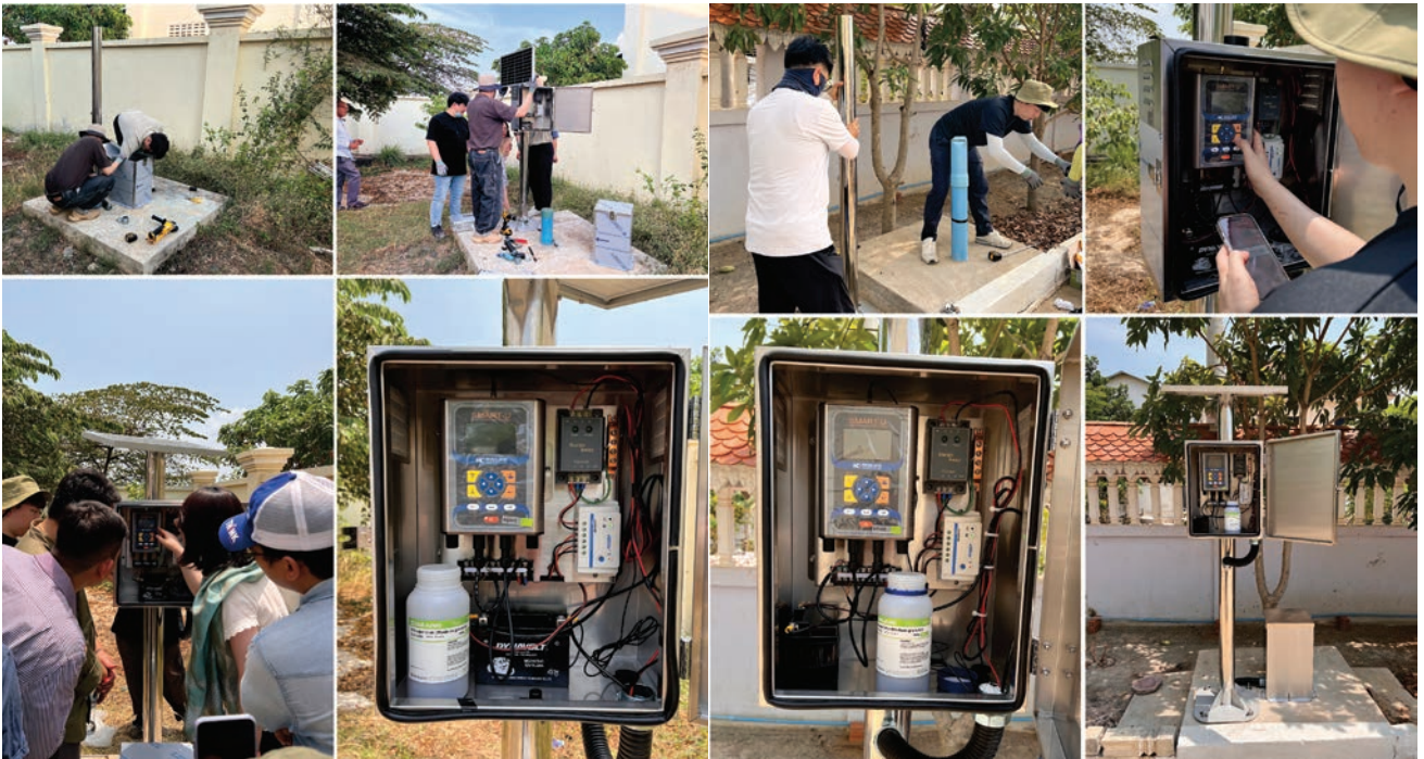
Groundwater monitoring system installation in Kampong in Cham Province, Cambodia
