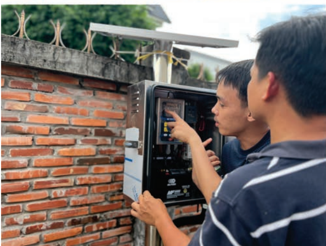
Groundwater monitoring system installation at Q209, Vinh Long Province, Vietnam
