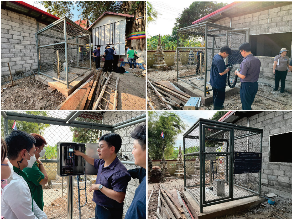
Groundwater monitoring system installation in Nong Khai province, North Thailand
