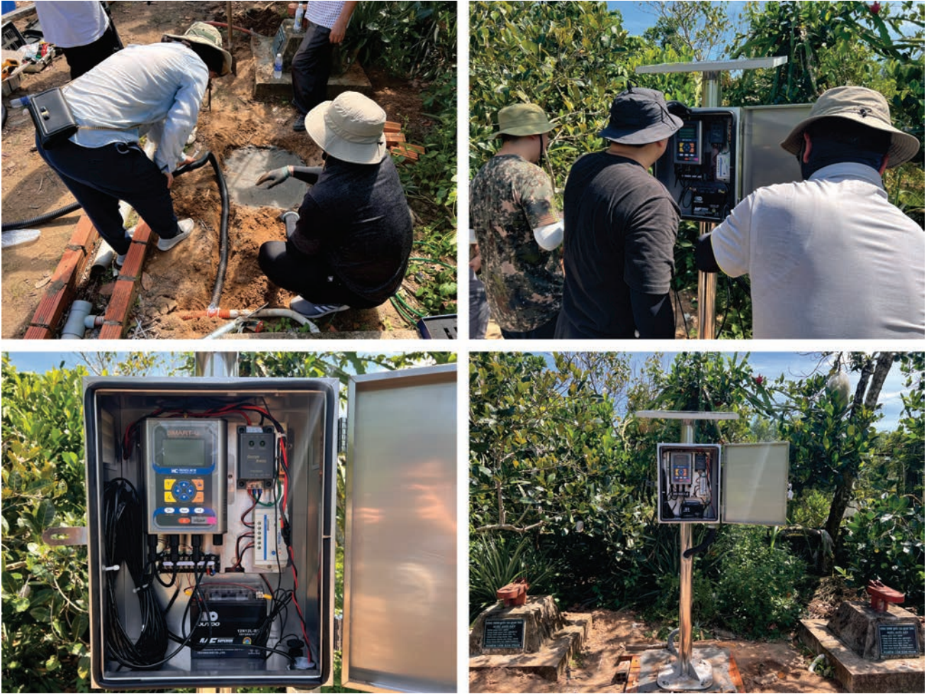
Groundwater monitoring system installation at Q606, Dong Thap Province, Vietnam
