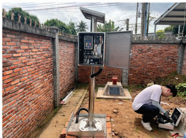
Groundwater monitoring system installation at Q209, Vinh Long Province, Vietnam
